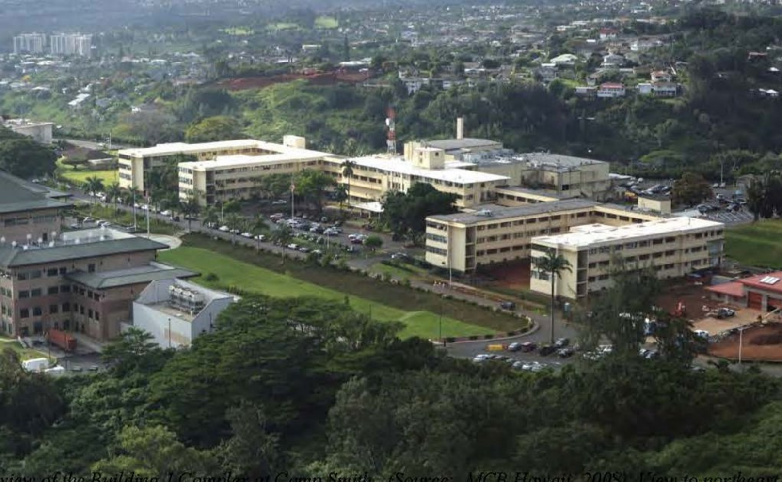
Enclosure 3: View of Building 1 Complex at Camp Smith Showing the Primary, South-Facing Façade fronting the Main Entry Road. Note: existing elevator machine room can be seen on the roof.
